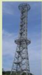
40m Toll tower
